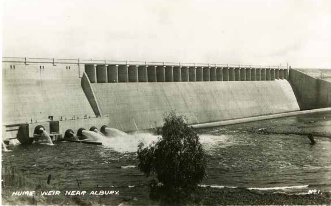
Fig. 1: Tourist photograph of Hume Dam, ca. 1940 ©by courtesy of AlburyCity Collections
